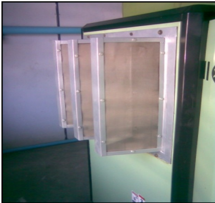
Fig 5. Pre-filter to existing Air intake Filter, pipe Extension to Air Entry. Fig 1. Invest in Air Receiver - / Tail End model
